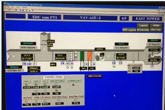
AHUs and VAV boxes
